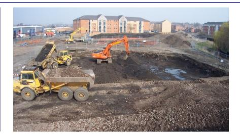
Remediation and Infrastructure works to a 3.6ha previous industrial site for development of student accommodation and commercial premises. The site has had a range of uses including; rail sidings, scrap yards, fuel depot, transport yard, garage and warehousing which has left a significant amount of hydrocarbon contamination (TPH) in the over-site fills.
